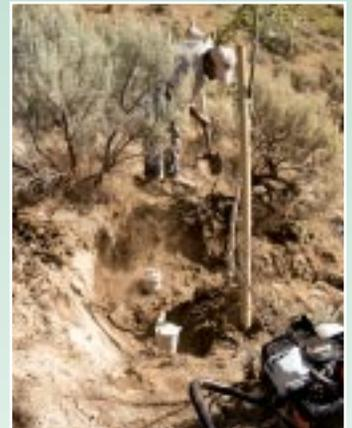
He immediately specified 1,250 Rain Bird RWS-BCG units with sand socks. Because of the sandy soil, he needed the units to encourage lateral root growth, so each RWS was cut to 24 inches. He also specified the sand socks to prevent the sand from infiltrating the RWS mesh tube.
